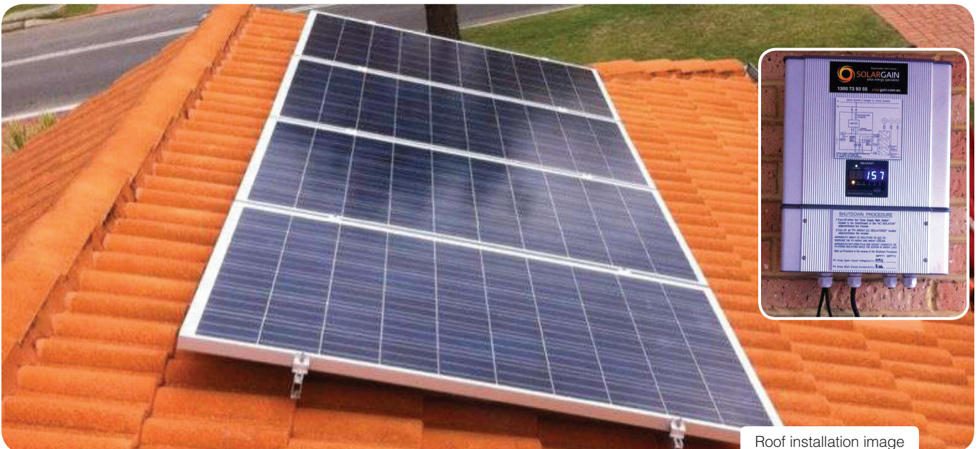
Roof installation image
