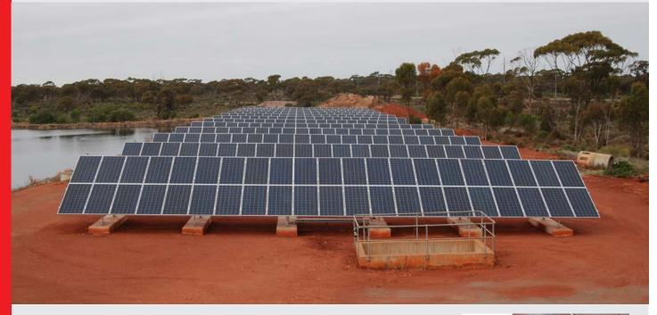
/ This 150kW PV installation in Western Australia provides power to the City of Kalgoorlie-Boulder's wastewater treatment plant. With a yearly energy production of approximately 273.5 MWh the system is estimated to provide cost savings of over \$60,000 per annum.
